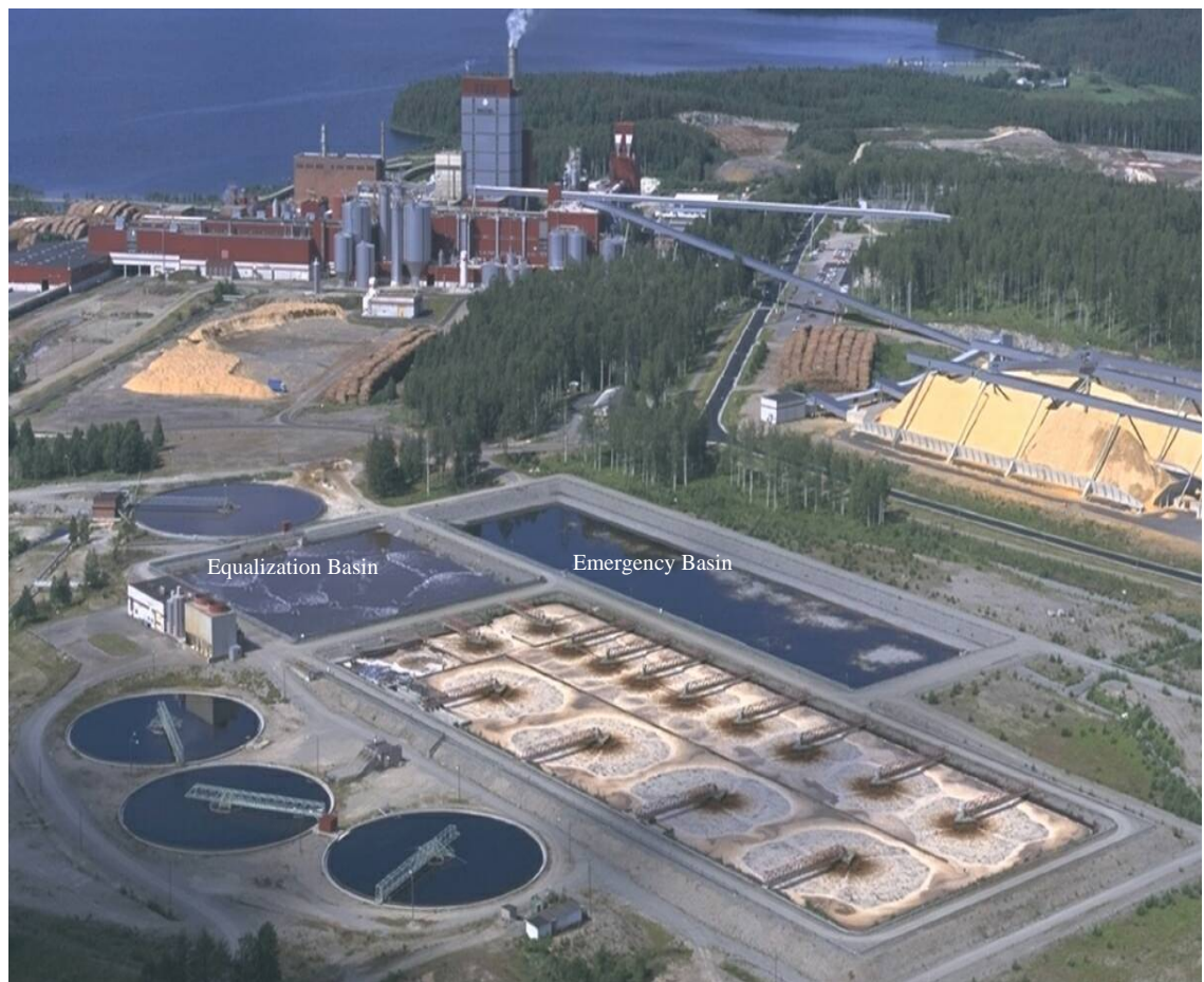
Figure 2/1. An Extended Aeration Activated Sludge Plant at a Pulp Mill in Finland
