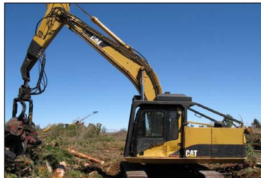
Excavator with cutting head
