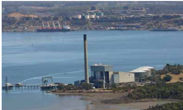
Figure 5.7.1: Power Station, north-west of the proposed site, on the bank of the Tamar River
