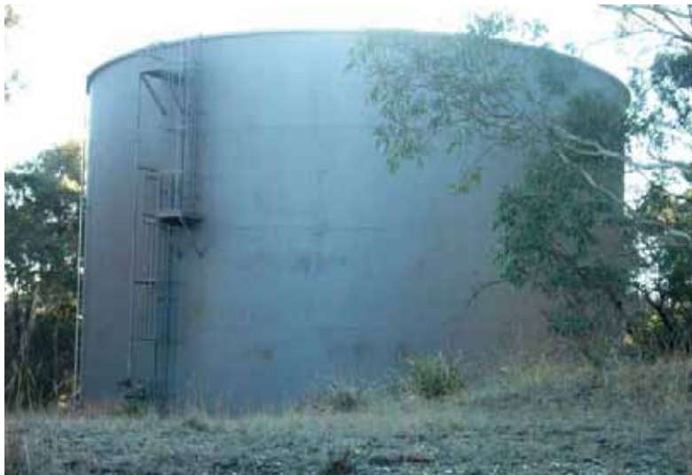
Photo 5.3.1: Water tank near access road to site
