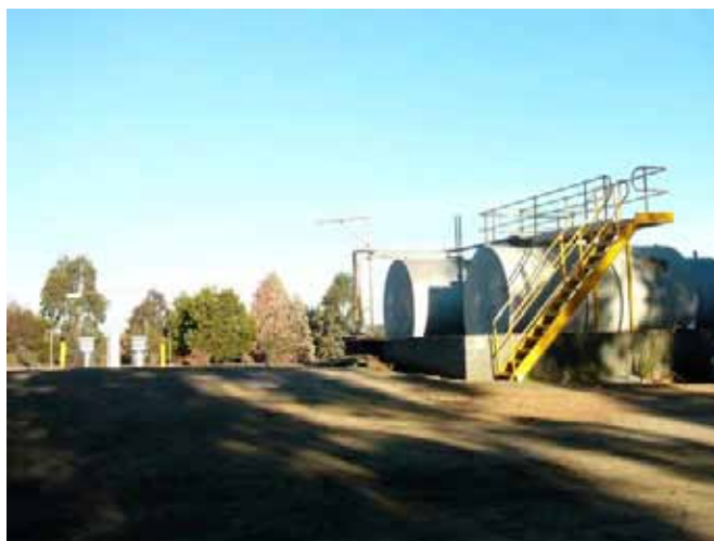
Photo 5.8.3: Fuel storage tanks, south-east of the proposed pulp mill site
