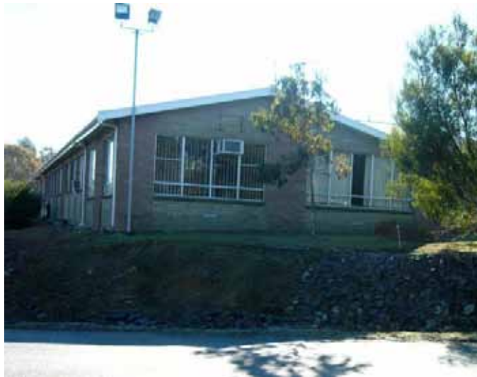
Photo 5.4.1: Upper level site office building
